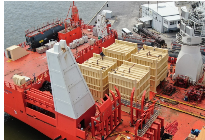
740 bbls tanks being installed
