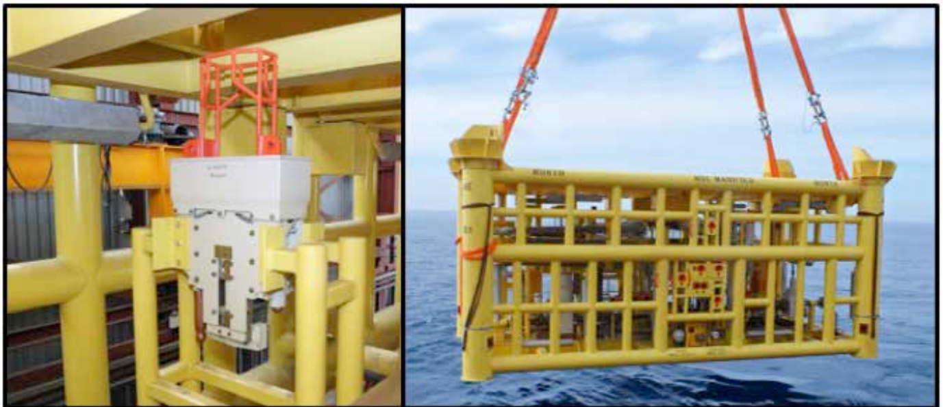
Figure 1: (Left) Preinstalled female connector on a manifold; (right) The manifold being deployed subsea.
